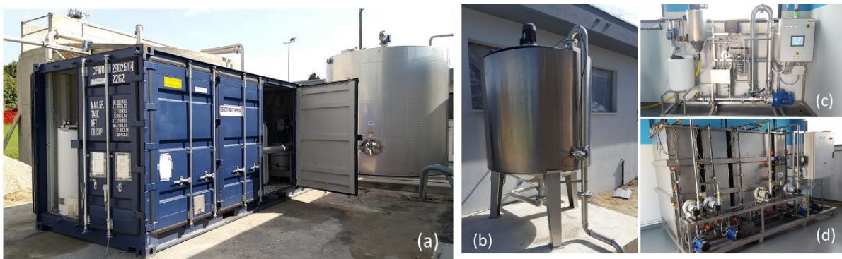
Figure 1 (a) Salsnes Filter SF1000 for the sieving of wastewater; (b) fermentation unit for the production of VFAs; (c) ceramic membrane for the solid/liquid separation and crystallizer for P-salts production; (d) Units in SBRs-modules for nitrification, PHA storing biomass selection and PHA accumulation.
